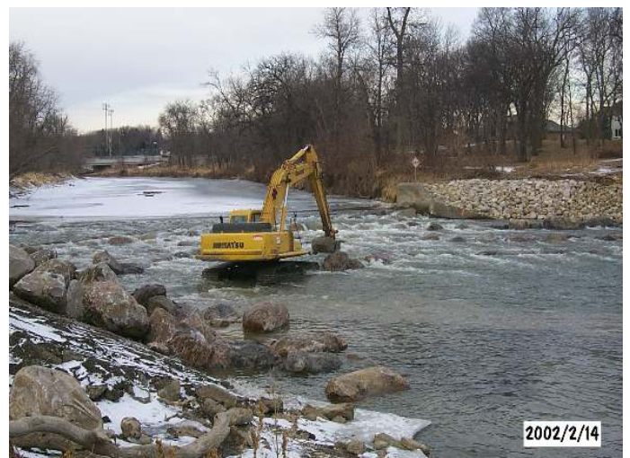
Placing the rocks for the dam retrofit in 2002.
