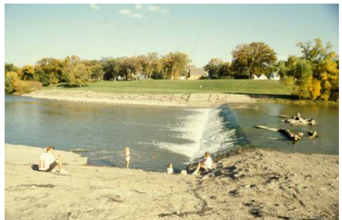
Midtown Dam before 1999.
