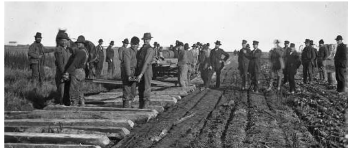
Workmen lay rails for the St. Paul, Minneapolis and Manitoba Railway, just east of Moorhead, 1880.
