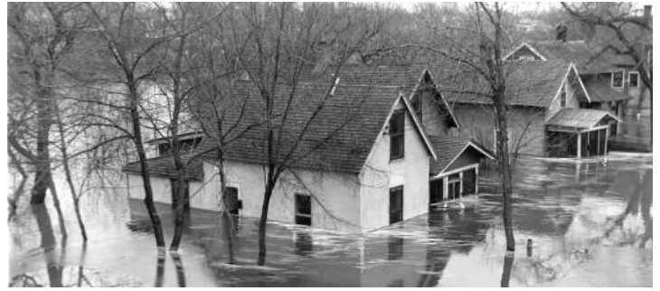
Flooded homes on the Point, 1943. The view is to the north from the 1 st Avenue North Bridge.
