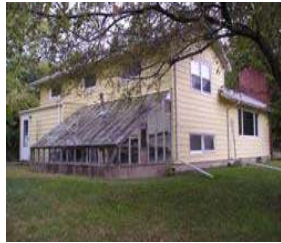
1. Existing House & Greenhouse
