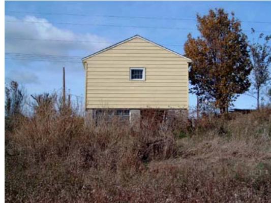
View of existing shed.
