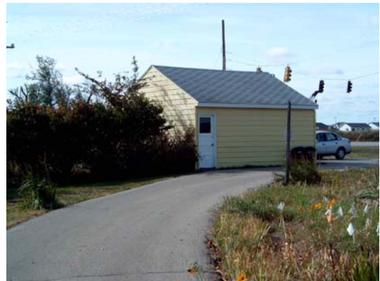
View of existing garage.
