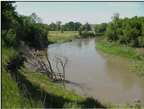
Rotational slump along Red River of the North in Fargo, North Dakota. Note the relationship of this activity to the cutbank and the outside of the river meander (left). (Photo by D.P. Schwert).
