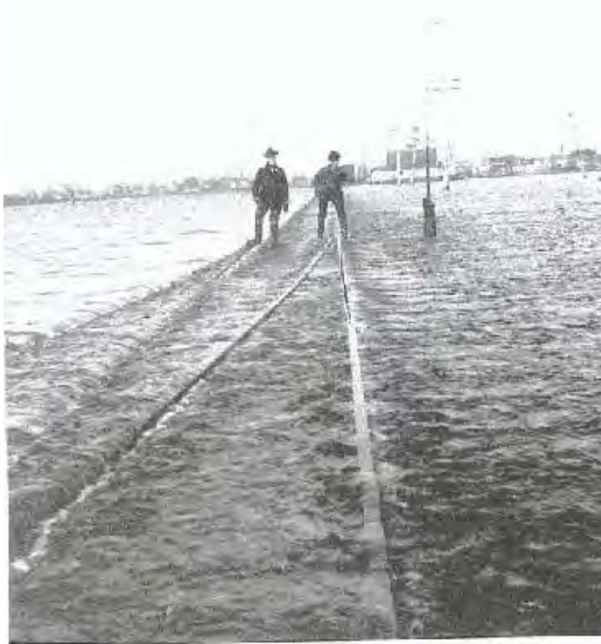
Great Northern tracks under water 1897-1898 Breckenridge, MN
